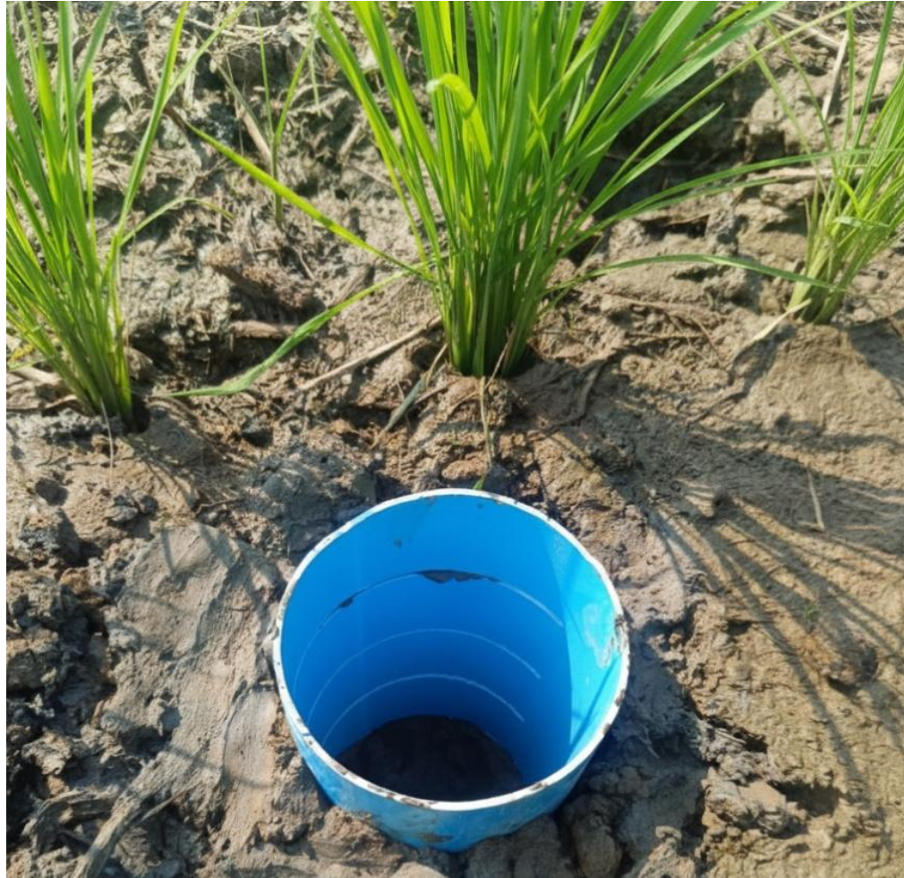
Figure 3: Installing perforated PVC pipe into the field to monitor the subsurface water level
