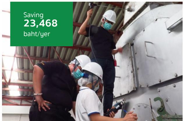
Project "Reduce excess air properly Increase efficiency burning of the boiler"
