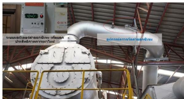
Oxygen Sensor for Monitoring Hot Water Boiler Combustion Efficiency
